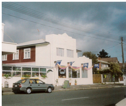
5 Commercial Road 1992 There was a real estate and garden centre here and no front verandah
