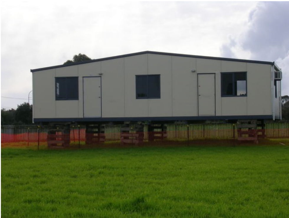
Modcom ready for siting, extension and completion
